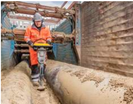
BS30 – The specialist for narrow trench applications and pipe gusset compaction.
