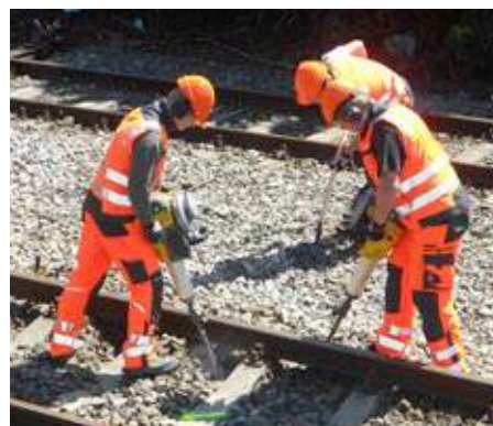
The gasoline hammers BH40 and BH55rw are optimally suited for maintenance works in the railway industry.
